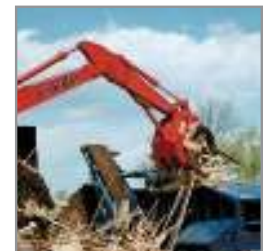
Wood Waste Handling
